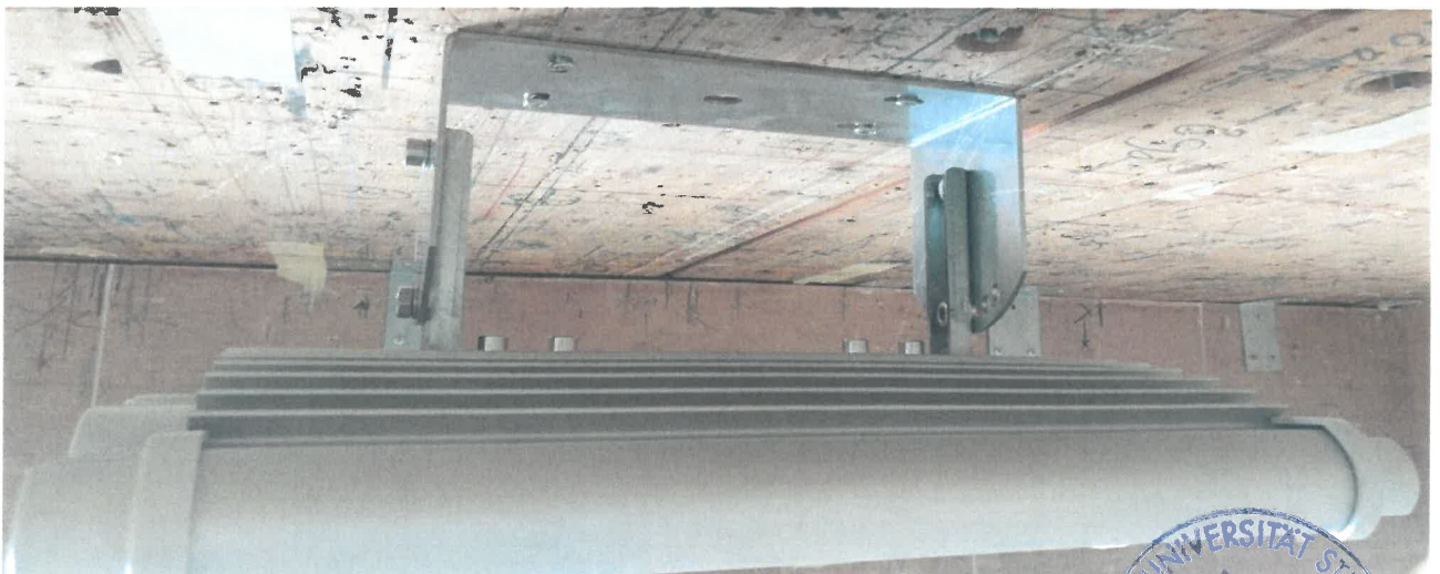
Picture 2 Detail: Suspension “H LUM (ST/PR.288)”
